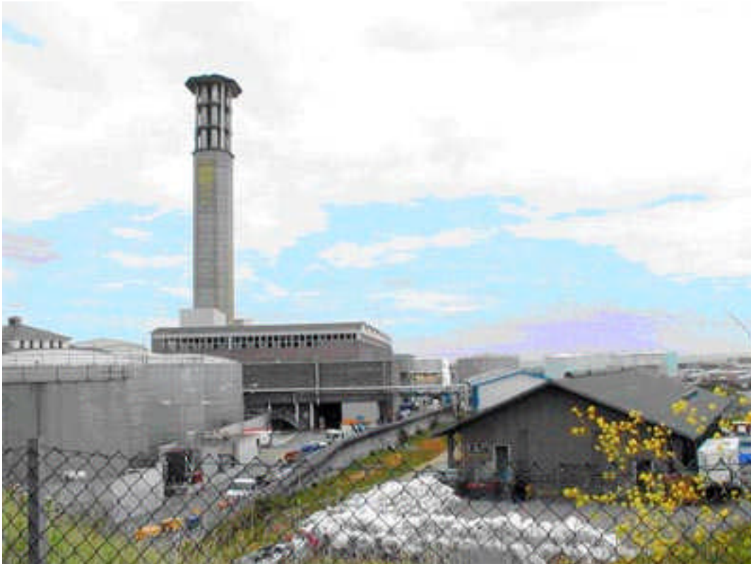
Photograph 2: The Jersey Electricity Company power station.
